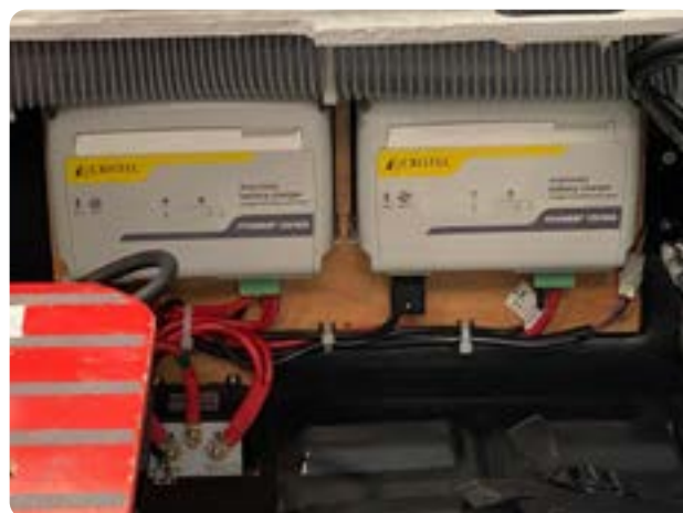
Cristec Y Power 12-40 charger installation
