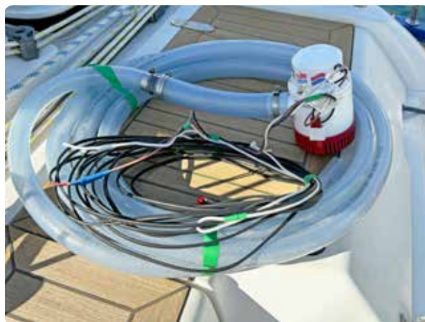
Emergency electrical pump with 233 litre/minute capacity
