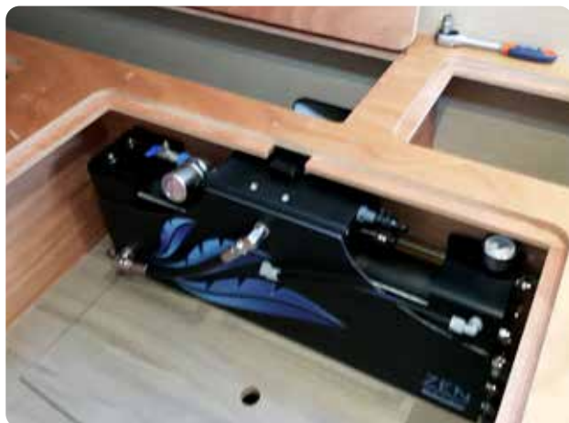
Schenker Zen 30 installed under a bunk
